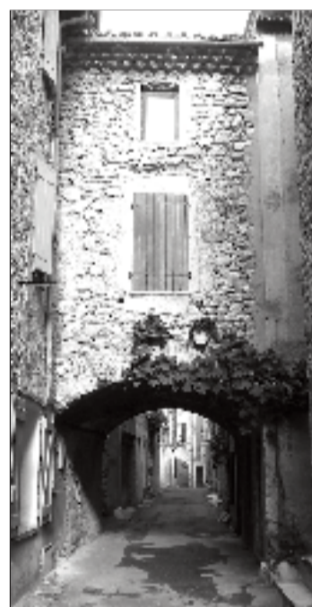
Stones from the river bed, reused ancient blocks, and quarried stone are the most common building materials. Roofs are covered with Roman tiles, and rimmed with rows of traditional “gênoises”. There are many engraved and carved lintels, stating the date when the house was built or renovated. You will also notice many old doorways and flying buttresses across the narrow streets.
